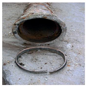
**Fig. 2.** In Philadelphia the joints of the pipes were filled with led, technique that was also used in Havana.
