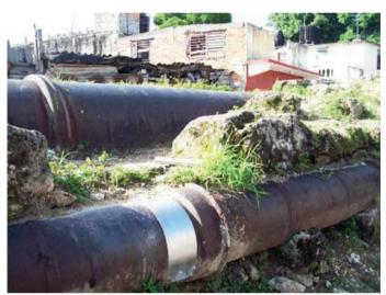
**Fig. 4**. Top to bottom: the iron pipes of Albear (1893) and Fernando VII (1835) showing a reparation. The pipes are on top of a wall built to protect them in the street named Resguardo (protection) in Cerro municipality.
